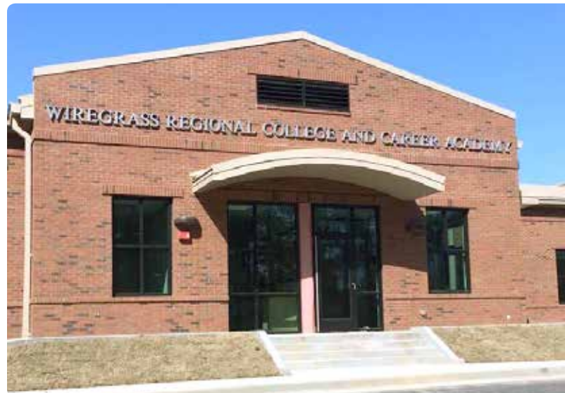
The new Wiregrass Regional College and Career Academy facility helps put students one step closer to preparedness for life after high school.
